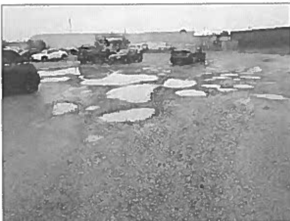
General view of the gravel surfaced parking areas noted on the north portion of the Site.
