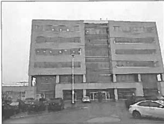
General view of the east elevation of the Site Building.
