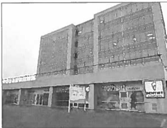
General view of the south elevation of the Site Building.
