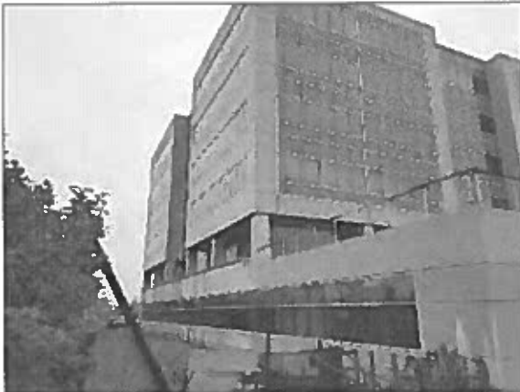
General view of the west elevation of the Site Building.
