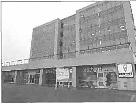
General view of exterior wall cladding of the Site Building.
