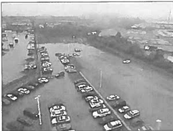
General view of the asphalt paved and gravel surfaced parking areas and driveways noted on the north portion of the Site.
