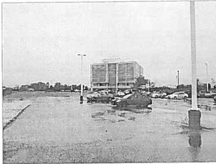
Photo 1 – Site Building (north elevation).
