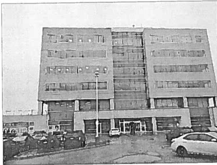
Photo 3 – Site Building (east elevation).
